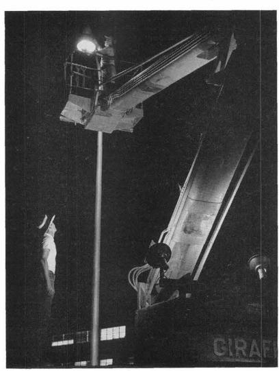
POWER HOIST called "The Giraffe" is used by B. A. Keller, left, and Louis Price, on platform, to install a new bulb in a street lamp near Bldg. 805. The men, both 4514-3, use the truck-mounted lift to maintain all outside lighting at Sandia Lab during non-working hours.
